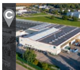
Location: Hartmannsdorf/Chemnitz Property: Lambda Transfer of ownership: 03/2022
